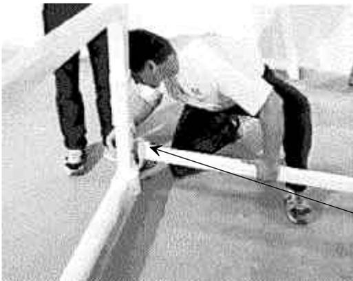
The *horizontal braces* are long rectangular tubing with L-shaped fittings welded to each end.
