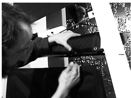
***Very important - Don't allow larger holds to overlap onto the next panel.*** The holds supplied with the Treadwall are designed so that they will not overlap, but other holds may be larger. Also, holds must not stick out more than 2 1/2" from surface of wall.
