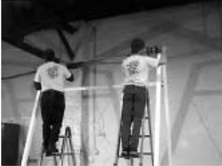
← □ **Raise the shaft to top of the frames.** Position the ladders slightly in front of the frames as shown. Line up the holes and place the mounting bolts with washers.
