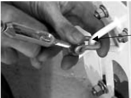
The *x-bracing* goes between the two channels - *turnbuckles* at the bottom.
