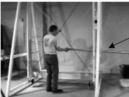
If there is an obstruction on the side where you are slipping in the pipe, you will have to move the assembly around for clearance.
