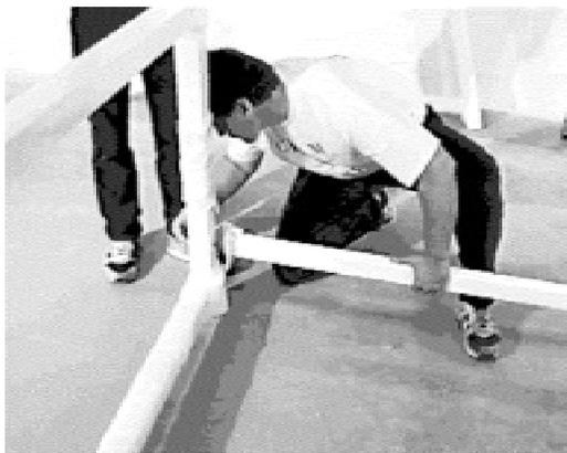
The *horizontal braces* are long rectangular tubing with L-shaped fittings welded to each end.
