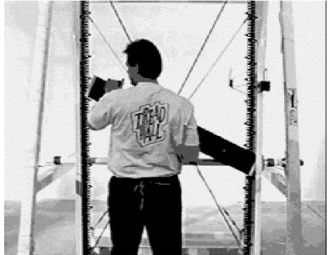
*Every second panel must be flipped end-for-end* so that the holes alternate.
