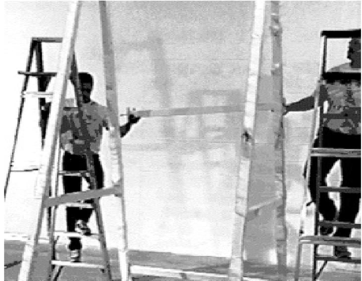
**Tension X-bracing** in the back makes the frame solid.
