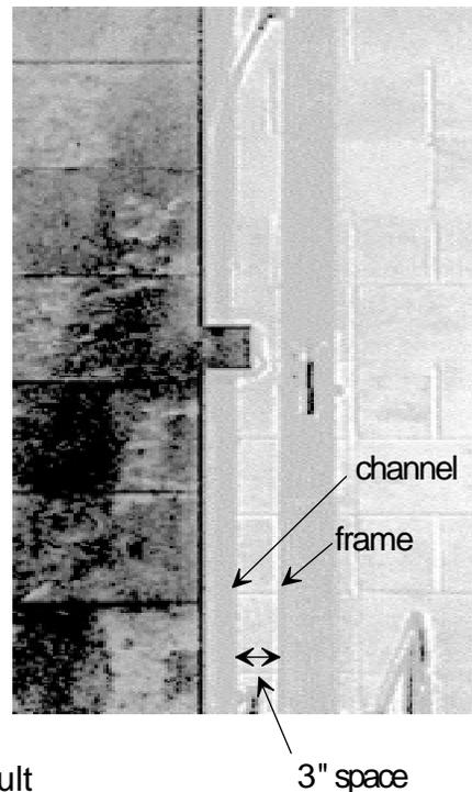
Handy-Tip: If this alignment is off, it may be difficult to lock the chrome ring on the adjuster pipe to the channel - the spacing will be wrong.
